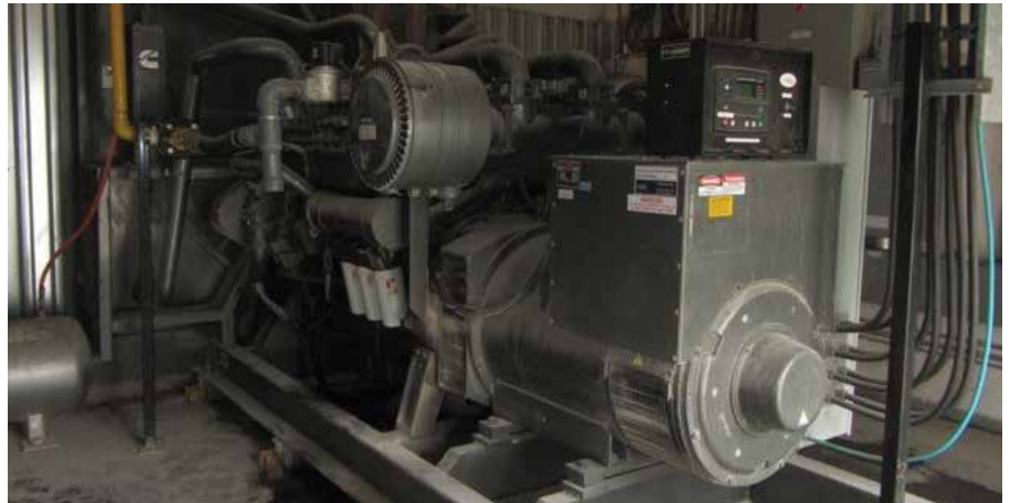
This large engine/generator (alternator) system effectively and efficiently powers a high throughput screen-less dryer.
