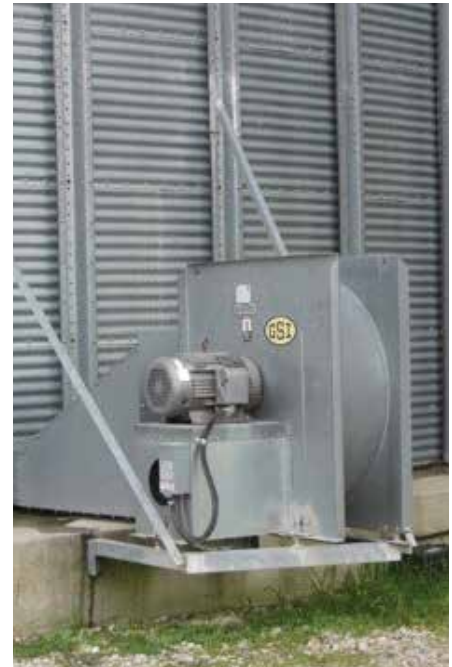
New large-diameter (high-capacity) grain bins require four 20-hp fans just for aeration to maintain the desired grain temperature.
