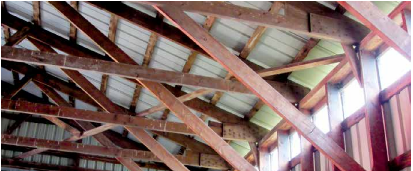
Many unlined farm buildings, such as machinery storage or loose housing livestock buildings, needed significant diagonal bracing for wind loading transfer.
